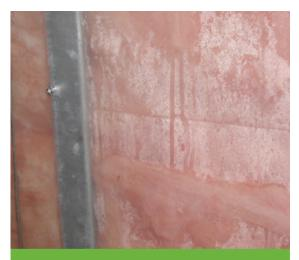
In the 1990's, air-conditioned homes with unventilated or poorly ventilated brick veneer were showing signs of condensation on the interior vapor barriers during the summer months. In the investigations that followed it was clear that the summer time condensation was in part due to reverse vapor drive.
