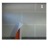
Begin installation at the base of the wall, progressing in a shingle fashion upwards.
