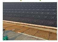
Standing Seam Metal Roof Optional use of VaproShim SA Self-Adhered under metal roof clips creates increased airflow under metal panels
