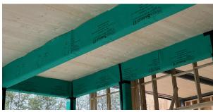
With a drying capacity of 123 perms, the framework dries out quickly and is less susceptible to ongoing wetting issues from weather events.
