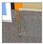
13. Install adjacent pieces of RSSA material. Pull mesh back and overlap WRB/AB a minimum of 3".
