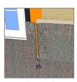
14. Overlap mesh from each side and cut at the same time vertically. Tack mesh in place with staples or hammer tacker.
