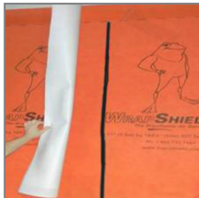
5. Apply VaproBond Adhesive Sealant in a single bead down the membrane to the bottom of the sheet.
