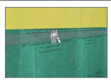
2. Install with SS staples in the top 2" above the Integrated Tape. Avoid stapling in the adhesive strip area of the Integrated Tape.
