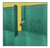
4. Overlap vertical seams by 12" minimum, seal with VaproLiqui-Flash or VaproBond Adhesive Sealant if necessary.
