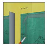
5. Remove release film from top of adhesive strip where flap overlaps.
