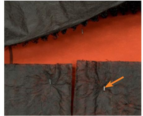
3. Mechanically fasten VaproMat approx. 2" down from the top edge with stainless steel (SS) staples. Continue securing VaproMat every 24".
