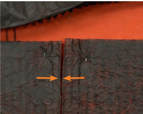
4. Vertical seams of VaproMat drainage matrix butt together and do not overlap.
