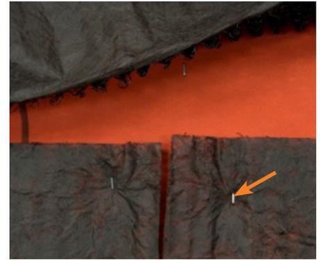
3. Mechanically fasten VaproMat approx. 2" down from the top edge with stainless steel (SS) staples. Continue securing VaproMat every 24". Remaining VaproMat material will be held in place by stone lathing fasteners.
