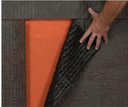
2. Place VaproMat horizontally against exterior wall, filter fabric side out. The drainage matrix should face the building interior. Starting at the bottom of the wall, position the first piece of VaproMat at the bottom edge of the stone where the weep screed is located (weep screed installed by others).
