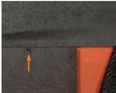
5. Horizontal seams of the drainage matrix butt together.
