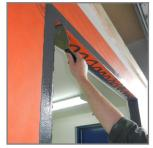
13. Immediately spread until all surfaces are completely covered and substrate below is no longer visible (approximately 12 to 15 wet mils).
