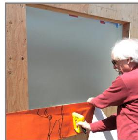
2. Install flashing at sill by minimally stapling it to the sheathing, leaving the lower 6" free for shingling over wall membrane.
