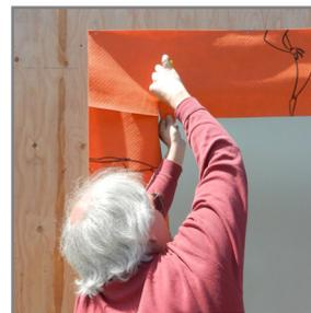
6. Using a sausage gun or DRY joint knife, apply VaproLiqui-Fash in a zigzag pattern on outer 2.75" of inside of rough opening.
