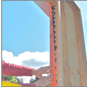
7. Immediately fold flaps into opening, pressing into the VaproLiqui-Flash with putty knife, spreading VaproLiqui-Flash evenly beneath WrapFlashing.
