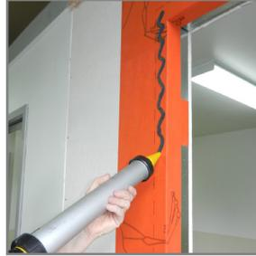
10. Using the sausage gun or DRY joint knife, apply VaproLiqui-Flash in a zigzag pattern on the wall face surrounding the rough opening.
