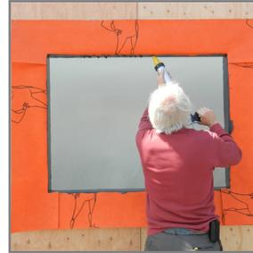
8. Using the sausage gun or DRY joint knife, apply a second layer of VaproLiqui-Flash over the folded flaps in a zigzag pattern on the inner surface of the rough opening.
