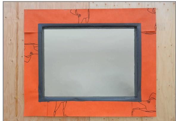
12. Allow VaproLiqui-Flash to set up until dry to the touch, then inspect for voids and apply additional VaproLiqui-Flash as needed to achieve complete coverage.
