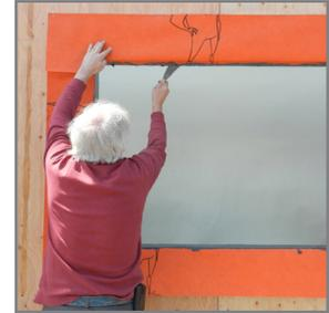
9. Immediately spread the applied material with a putty knife, fully embedding the inner flaps of WrapFlashing sill, right & left jamb, and head pieces, fully covering all inner surfaces of rough opening.
