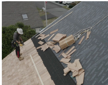
Cedar Shingles/Shakes With VaproMat™ Drainage Matrix
