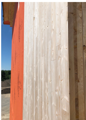
Figure 2-5 (Above) Small gaps between CLT laminations may not be completely airtight, thus requiring a separate air barrier membrane.
