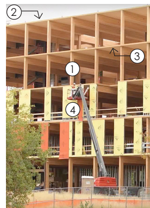
Figure 2-2 (Above) Mass timber building under construction.
