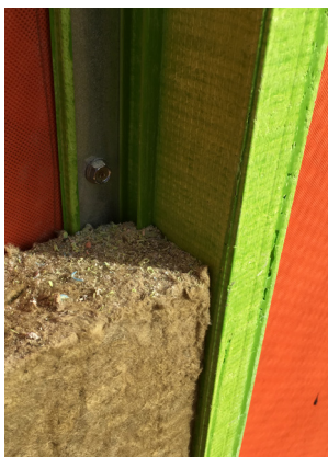
Figure 2-6 (Above) Photo of mineral fiber insulation installation being installed between vertically oriented fiberglass girts.
