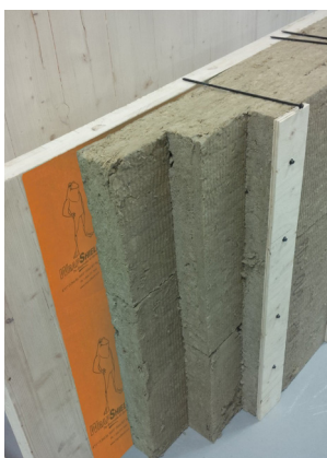
Figure 2-7 (Above) Vertical wood furring with long-screw fastener attachments and rigid mineral fiber insulation installed over VaproShield WrapShield SA Self-Adhered/CLT.
