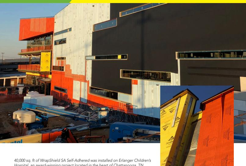
40,000 sq. ft of WrapShield SA Self-Adhered was installed on Erlanger Children's Hospital, an award-winning project located in the heart of Chattanooga, TN. The \$45 Million-dollar structure features a high-performance building envelope assembly consisting of multiple substrates, VaproShield WRB/Air Barrier solutions, exterior rigid insulation, and façade materials.
