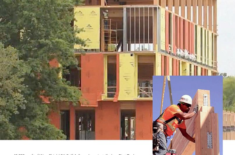
40,000 sq. ft of WrapShield SA Self-Adhered was installed on First Tech Credit Union, the largest documented U.S. building to use cross-laminated timber (CLT). The 156,000-square-foot building consists of glulam beams and CLT with a steel brace frame lateral restraint system.
