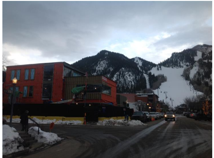
WrapShield SA Self-Adhered Water Resistive Vapor Permeable Air Barrier Sheet Membrane (orange) was installed over gypsum sheathing and FRT plywood—its adhesive bonds directly to virtually all substrates
