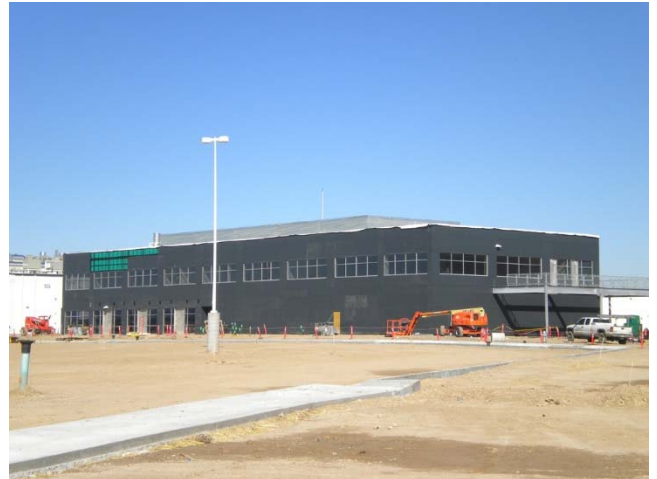
Largest wind tower manufacturing facility in the world.
