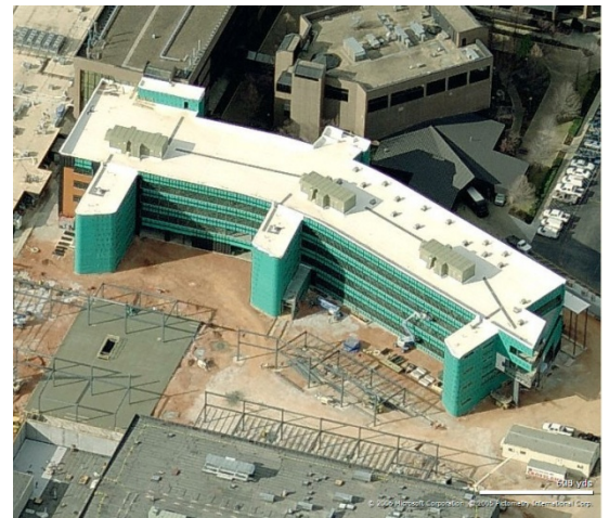
Aerial view of project with WallShield installation complete
