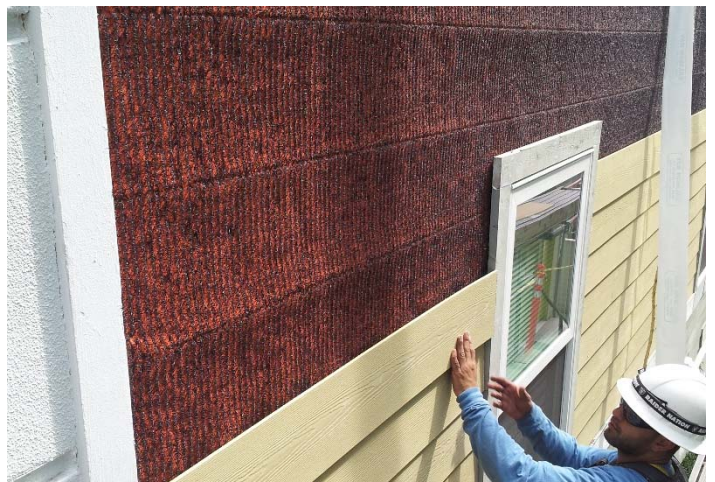
One step rain screen cavity installation with WrapShield RS saved $1.00 per sq. ft. vs. traditional batten rain screen systems.
