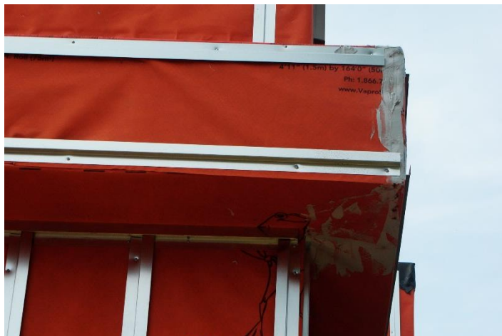
WrapShield with Integrated Tape at horizontal seams eliminated water concerns at horizontal joints and can be installed in all weather conditions.
