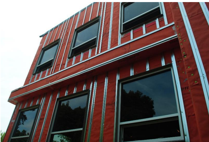
VaproFlashing Window Flashing Elements are manufactured using VaproShield's patented breathable membrane fabric, using an ultrasonic welding process, eliminating weak joints. They protect against moisture intrusion and entrapment around windows and doors.
