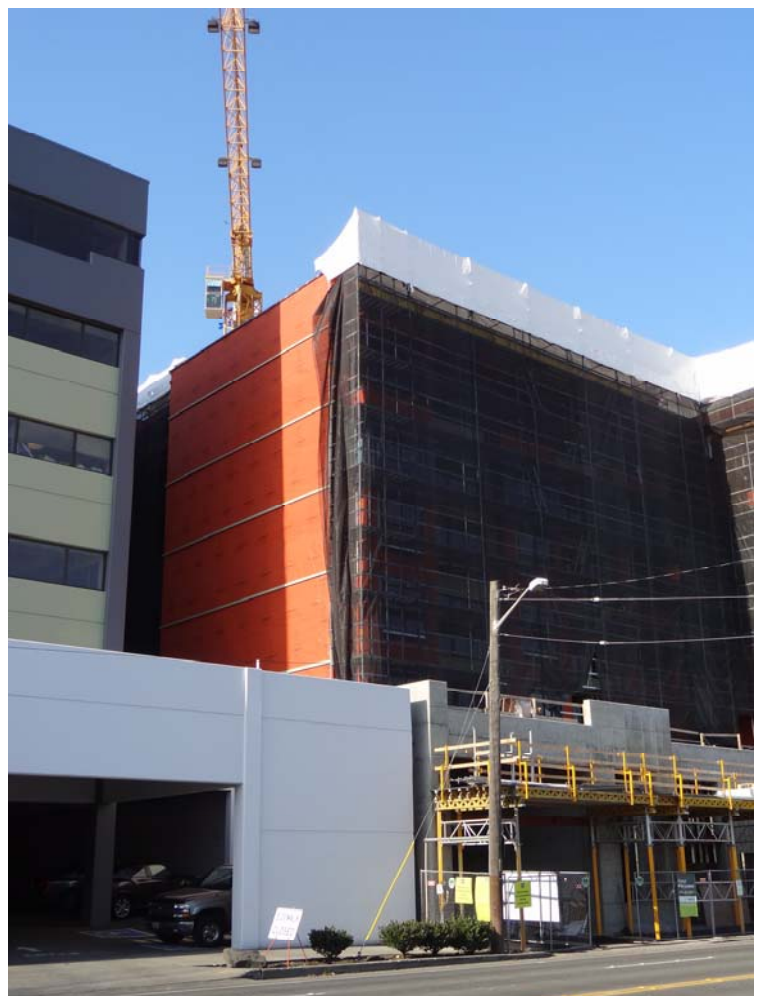
WrapShield helps to protect the True North apartment complex's delicate building envelope by reducing moisture intrusion and preventing mold, mildew and rot.
