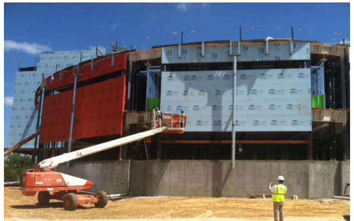
WrapShield SA Self-Adhered was installed over Dow Thermax CI insulation.
