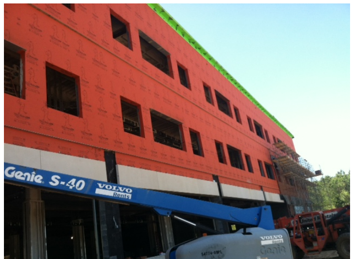
WrapShield SA Self-Adhered was installed over Dow Thermax CI insulation.
