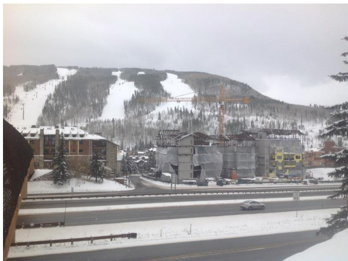
Over 60,000 sq.ft. of WrapShield SA Self-Adhered was installed behind multiple cladding types including copper, stucco, natural cedar and stone during the winter months.
