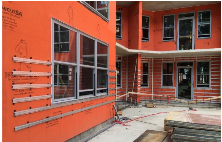
VaproShims used under horizontal cladding attachment components create a small, effective ¼" rain screen cavity, allowing for unimpeded vertical drainage of moisture away from the building envelope.
