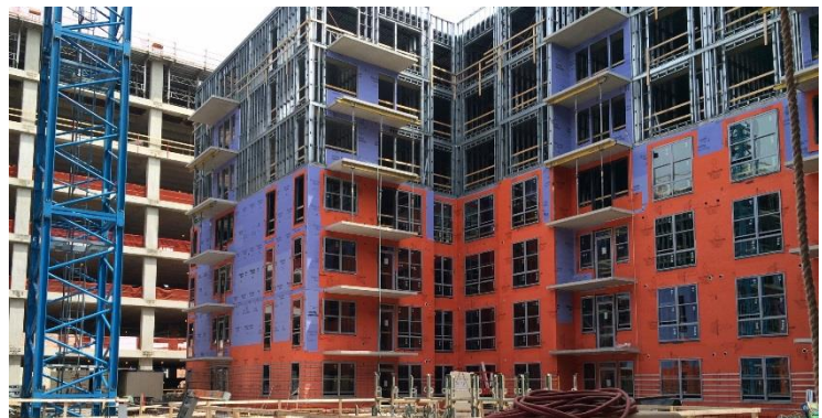
WrapShield SA Self-Adhered is applicable for all climates and weather conditions, and can be installed in temperatures as low as 20°F (-6° C)
