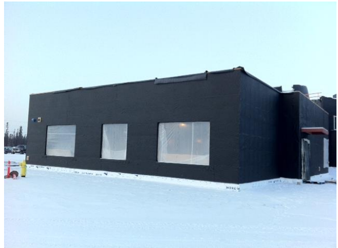
WallShield acts as the long-term water proofing layer.
