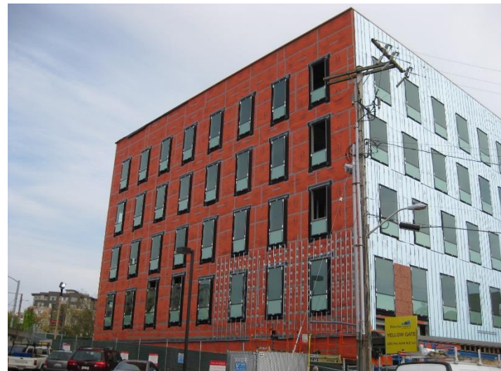
WrapShield, used as an air barrier, ensures no mold development in the wall cavities.
