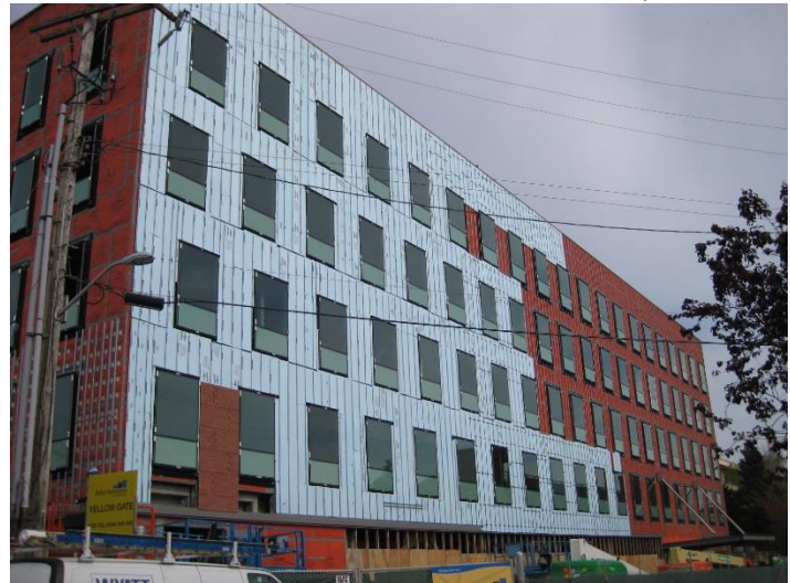
WrapShield, used as an air barrier, ensures no mold development in the wall cavities.
