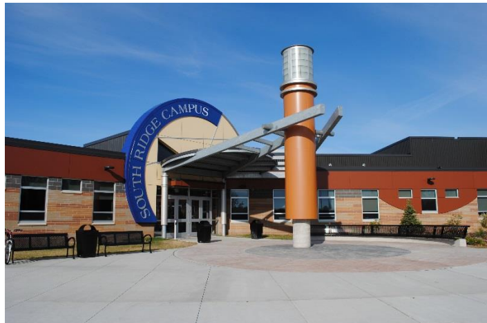
WrapShield Water Resistive Vapor Permeable Air Barrier Membrane was installed on the South Ridge Campus of St. Louis County Schools.
