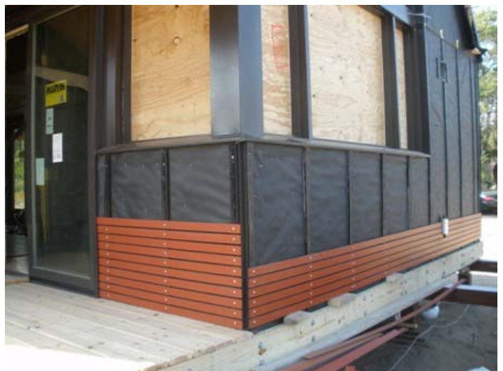
Close up of windows using VaproTape, VaproFlashing and 3D corners..
