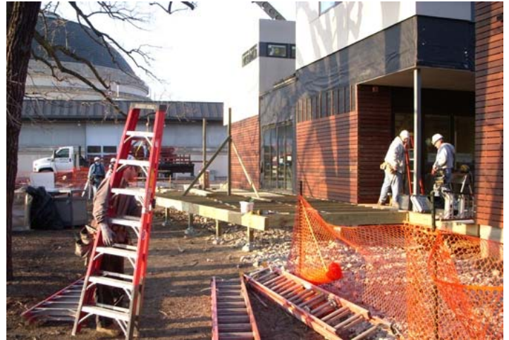
Black WallShield under the open joint rain screen design cladding.
