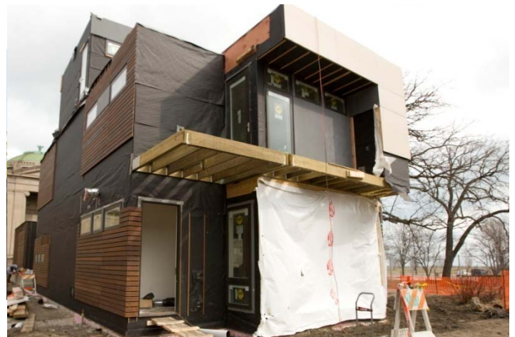
Pre-fabricated units installation.
