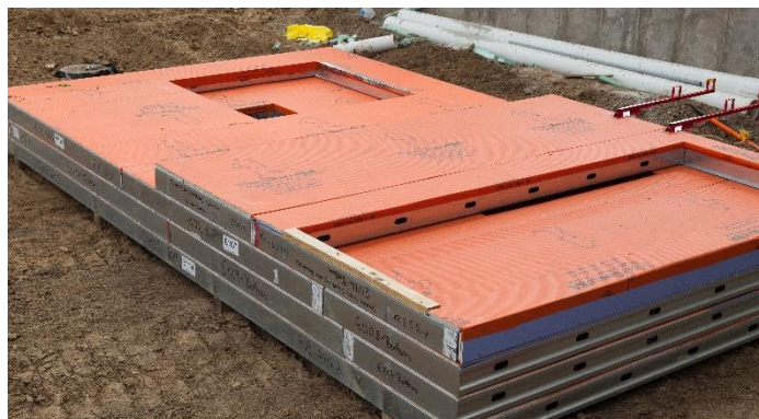
The panelized construction began in North Carolina where WrapShield SA Self-Adhered was installed to the sheathing and then shipped to Lansing.
