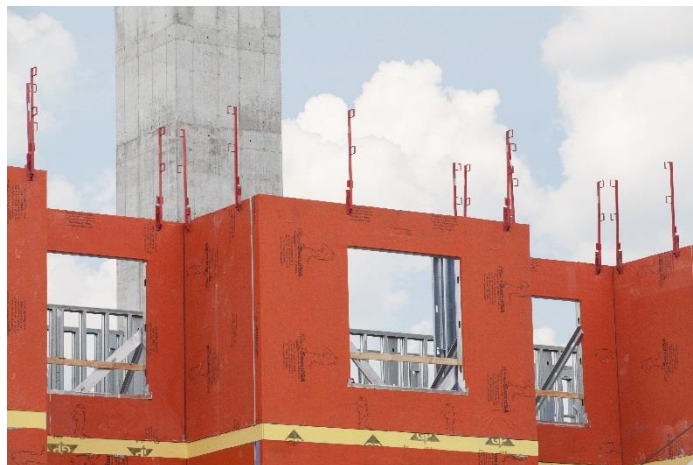
The panelized construction began in North Carolina where WrapShield SA Self-Adhered was installed to the sheathing and then shipped to Lansing.
