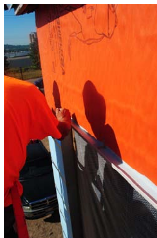
WrapShield SA Self-Adhered is tough, durable and tear resistant during installation. It can be applied temperatures over 20°F (-6°C) and rising.
