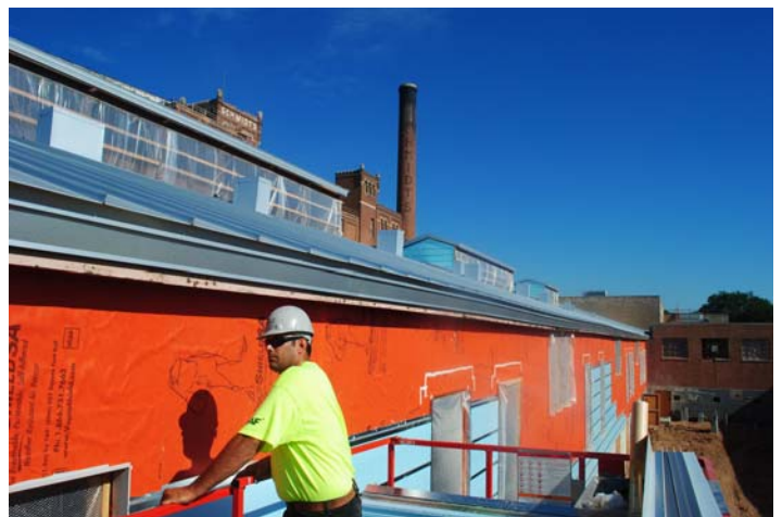
WrapShield SA Self-Adhered is tough, durable and tear resistant during installation. It can be applied temperatures over 20°F (-6°C) and rising.
