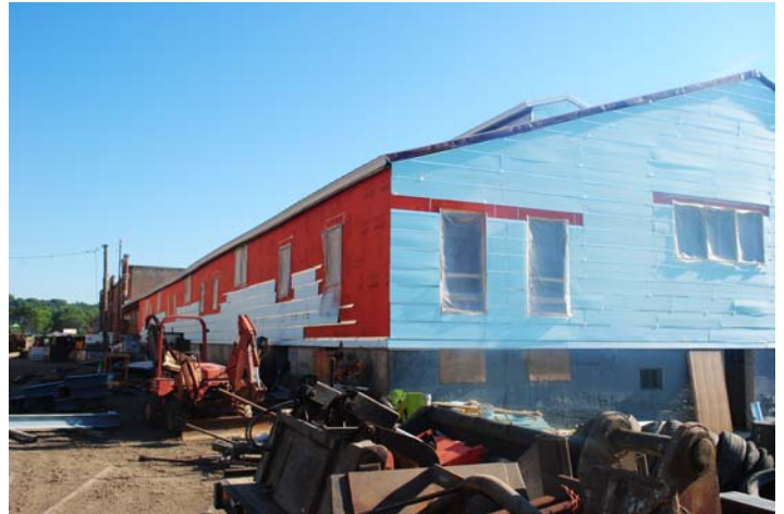
Over 15,000 sq. ft. of WrapShield SA Self-Adhered was installed on the restoration of the Old Schmidt Brewery.
