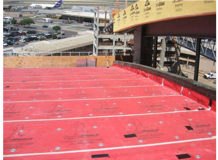
Over 90,000 Sq.Ft. of SlopeShield Water Resistive, Vapor Permeable Roof Underlayment was used on the new terminal.
