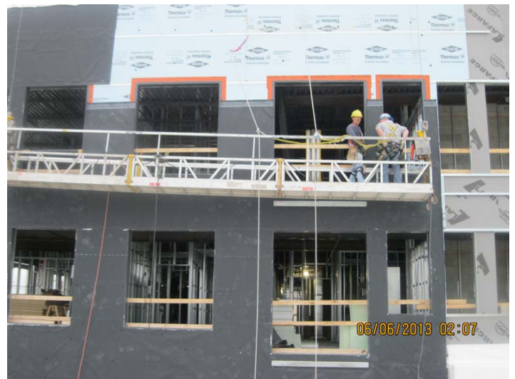
RevealFlashing Pre-Cut Flashing Membrane and VaproLiqui-Flash components were used to flash window and door rough openings.
