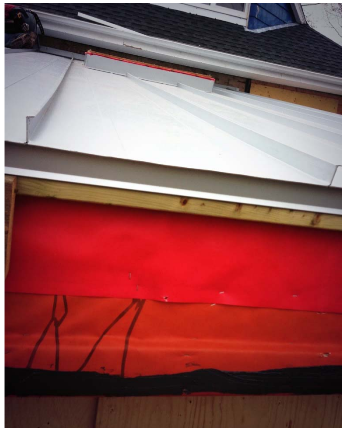
Both WrapShield Water Resistive Vapor Permeable Air Barrier and SlopeShield Water Resistive Roof Underlayment were used on the renovation project.
