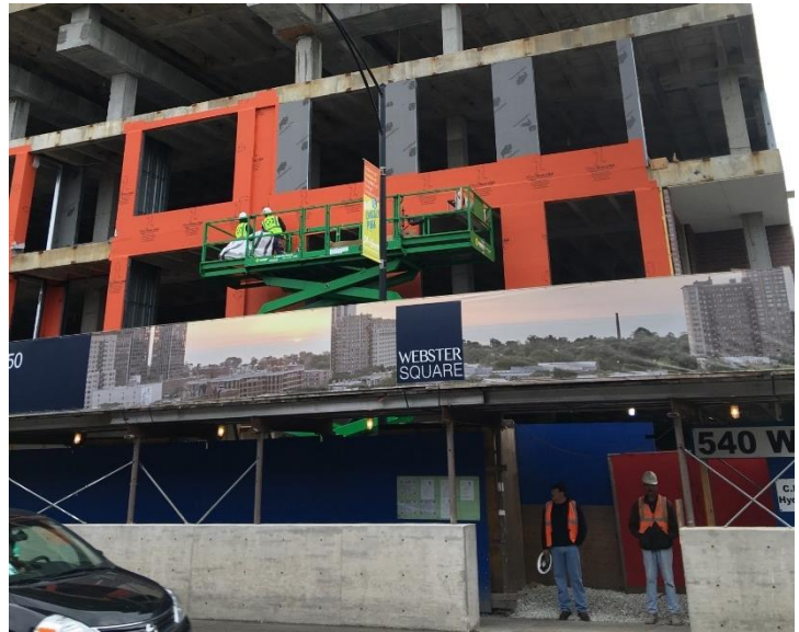
WrapShield SA Self-Adhered WRB/Air Barrier (orange) was installed on the Webster Square Condos in Chicago, IL.
