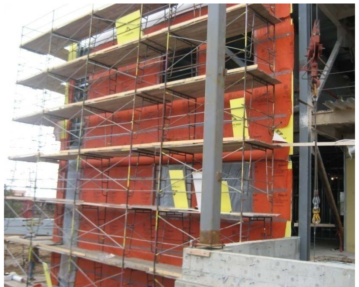
WrapShield installation progress
