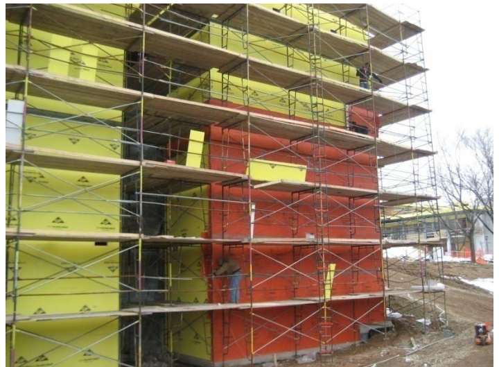
Early stages of WrapShield (orange) installation
