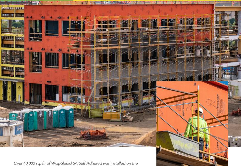
Over 40,000 sq. ft. of WrapShield SA Self-Adhered was installed on the Viega LLC headquarters in Broomfield, CO. The innovative building features a structural system of cross laminated timber (CLT), a renewable woodbased material that is quickly gaining market traction due to its strength, versatility, and sustainability.
