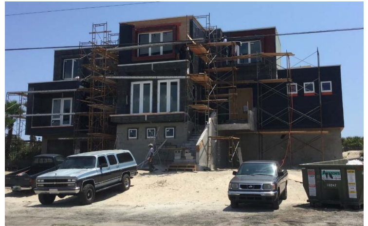
Two types of cladding were used: stucco and open joint rain screen cladding. WrapShield RS 7mm and RevealShield provided a single source solution including window flashing products.
