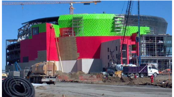
Over 150,000 sq.ft. of WrapShield SA Self-Adhered Water Resistive Vapor Permeable Air Barrier Sheet being installed in a special color: red to match Cornhusker red.
