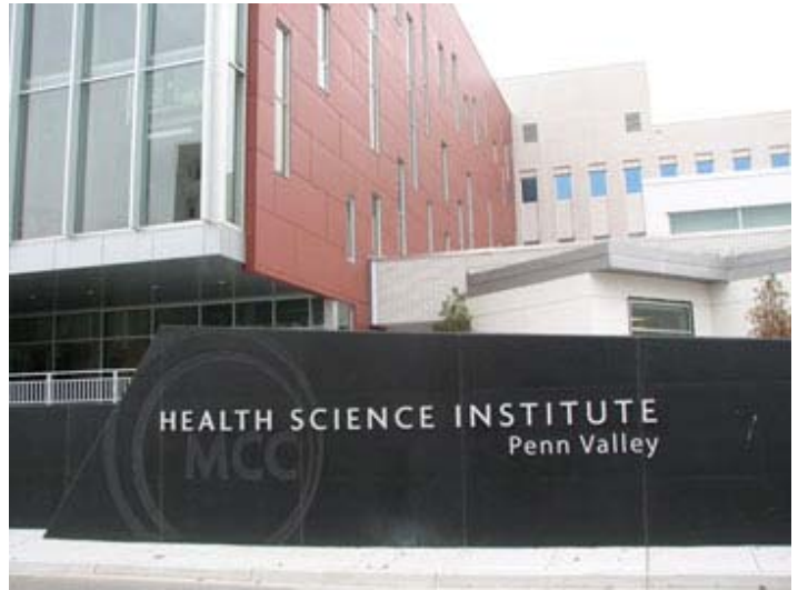
WallShield Black was installed on the new Health Science Institute.
