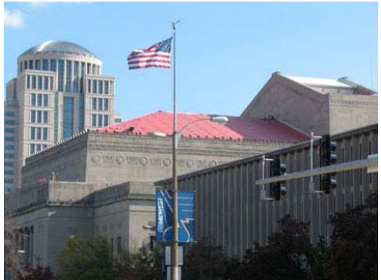
Installed under the roof material is 30,000 sq.ft. of SlopeShield Water Resistive Roof Underlayment, protecting the historic structure.
