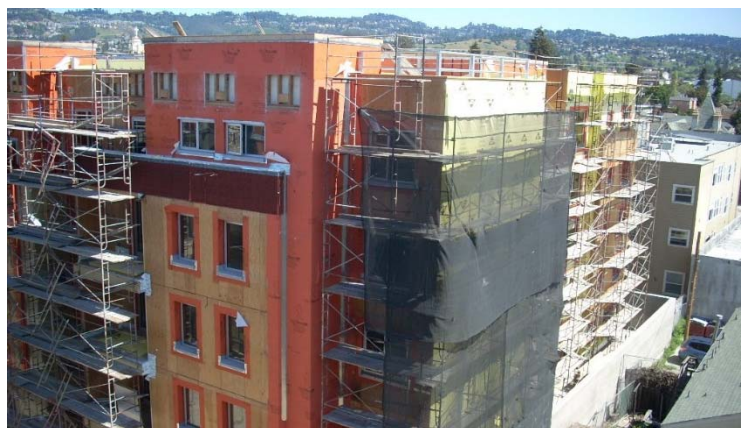
WrapShield RS Rain Screen offers a one-step installation of WRB, air barrier and rain screen cavity.
