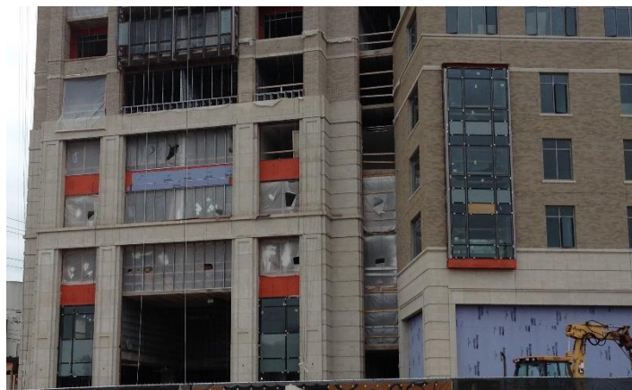
Tear, rip and puncture resistant during and after construction, WrapShield SA reduces repairs and labor costs.
