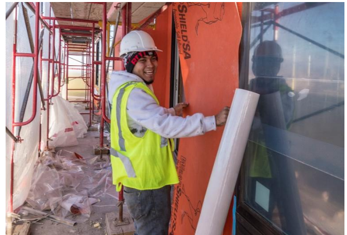
WrapShield SA Self-Adhered does not require harmful primer; crews are safe around the membrane and application was done with less labor.
