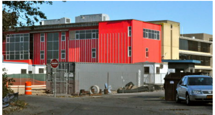
WrapShield SA Self-Adhered air barrier remained intact in torrential rainfall and wind gusts of over 70 mph. Source: LongBeach.Patch.com
