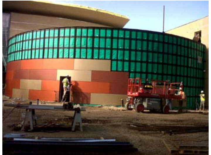
WallShield, along with VaproFlashing Black, were used behind open-joint Trespa TS 110.
