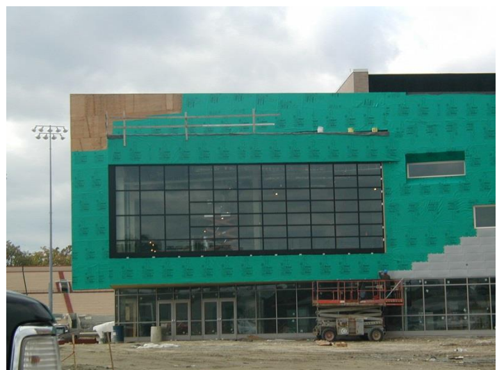
WallShield was installed behind the Rheinzink exterior cladding.
