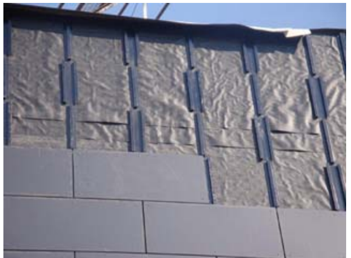
2000 s/f of WrapShielded Black was installed behind Trespa Meteon.
