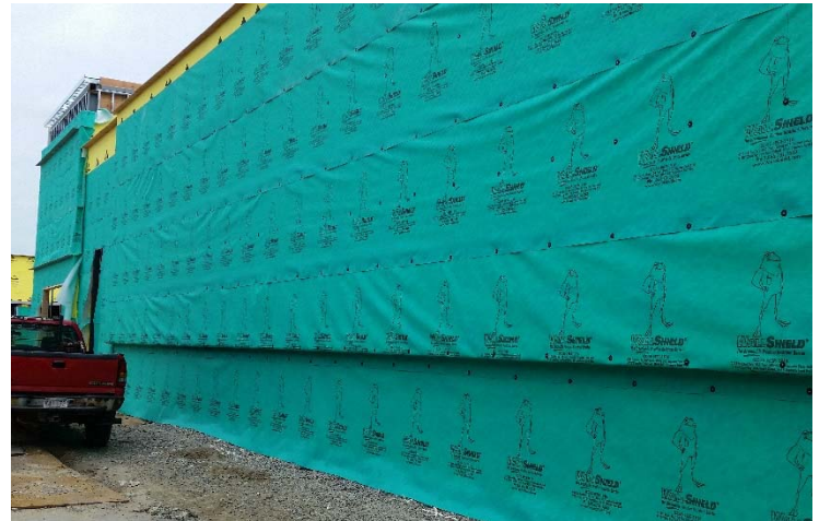
WallShield Water-Resistive Barrier Membrane allows any consequential moisture in the wall system to breathe out.
