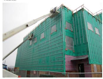
Rain Screen Design and 3D Flashing Elements were used during the installation of WallShield.
