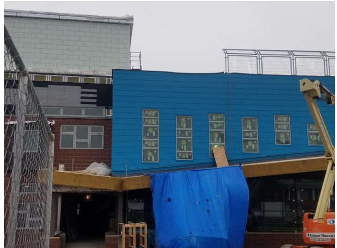
RevealShield IT Integrated Tape was installed to protect the mineral wool from wind and water infiltration, allowing it to maintain its intended R-value.
