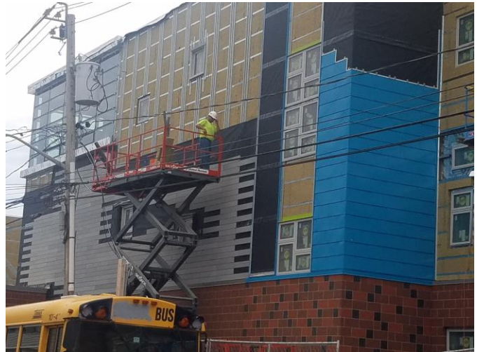
RevealShield IT Integrated Tape was installed to protect the mineral wool from wind and water infiltration, allowing it to maintain its intended R-value.
